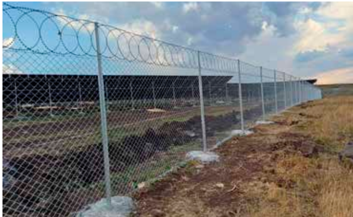
2 Rows of Barbed Wire Application Above 1.20 m Fence
