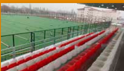
16 SPORTS FACILITY CONSTRUCTION
